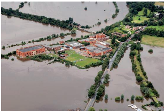
Figuur 9-7 Ondergelopen pompstation, Mythe, Gloucestershire, VK, 2007 (bron: Sinisi and Aergeerts 2010)
