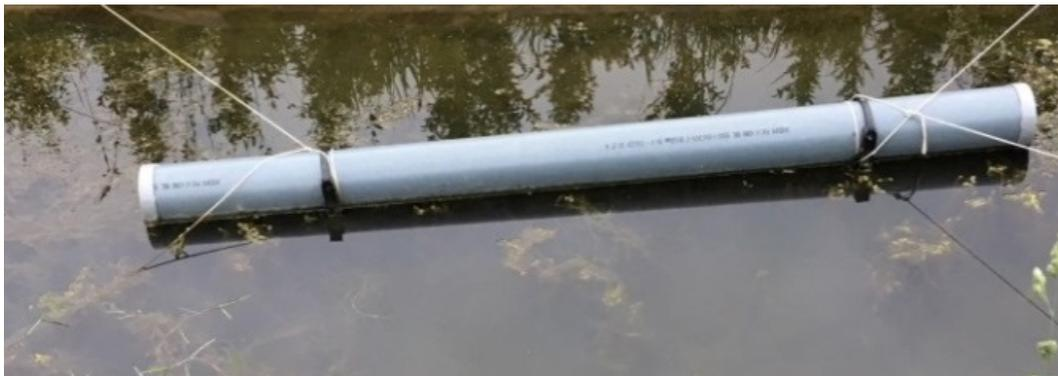
**Figure 4-33: Galileo L filter inlet during normal conditions (19-6-2018)**
