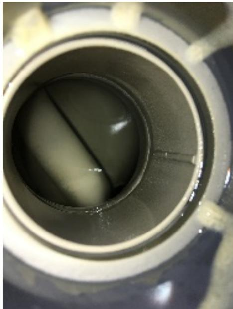
**Figure 5-3:** Inside the V-140 UV unit. The UV lamp is covered with mineral scaling (probably calcium carbonate)
