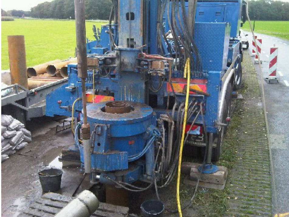
Drilling at Helvoirt
