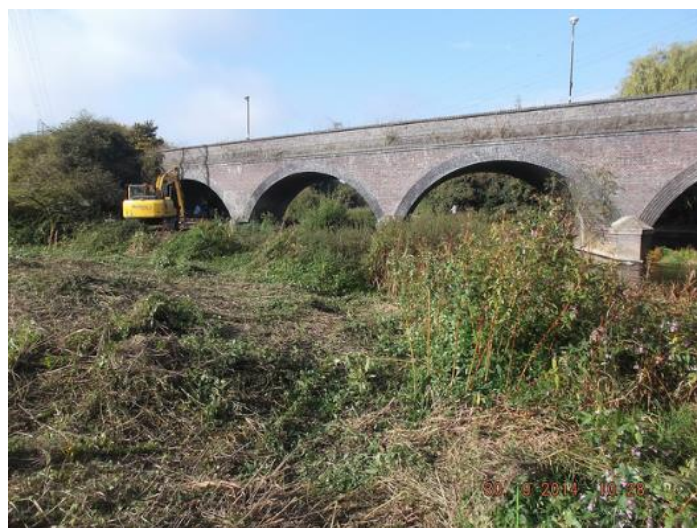
Figure 3 Increasing river flow capacity at the Great Central Way Biam Bridge.
