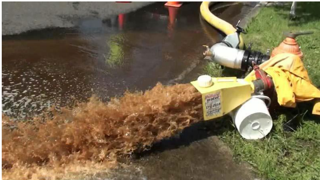
Figure 64 Pipe flushing operation.
