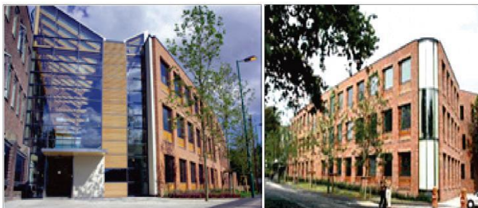
Figure 39 Administration and Student Services Building, University of Southampton (Rainharvesting systems 2012).
