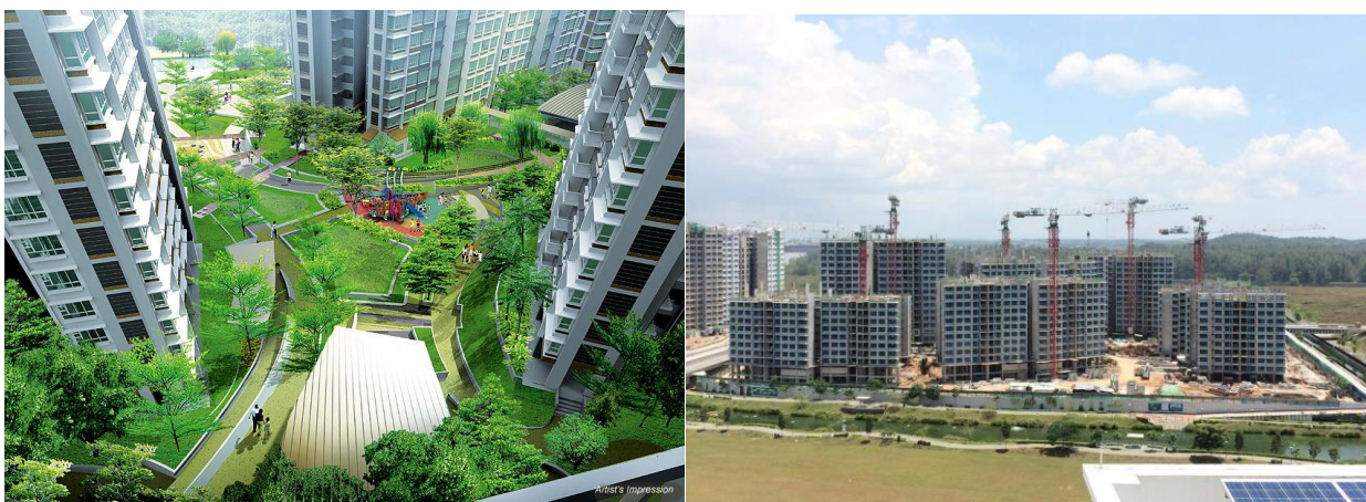
Figure 19 Design and construction of Punggol waterways ridges in Singapore. These ridges are rainwater detentions that form a train of water gardens and swales in which stormwater runoff infiltrates.
