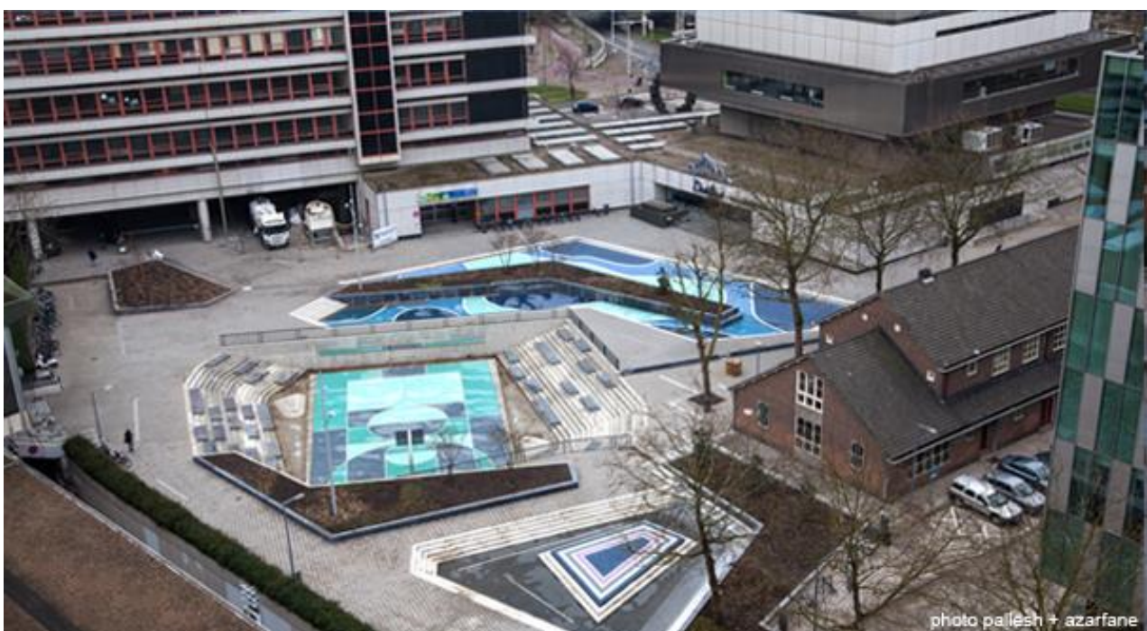
Figure 18 Water square Benthemplein, Rotterdam (Rotterdam Climate Proof 2017).
