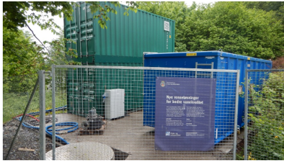
Hoffselva partners install the container with cross-flow lamella settler
