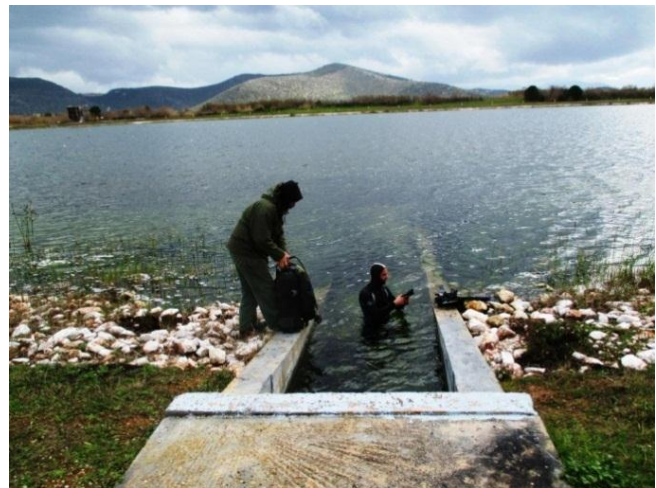
Figure 21. Installation of water pipes and power cables through the canal by divers
