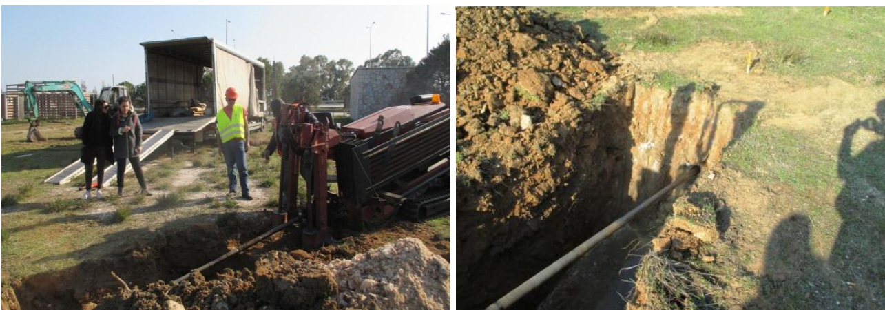
Figure 38. Horizontal Directional Drilling well construction
