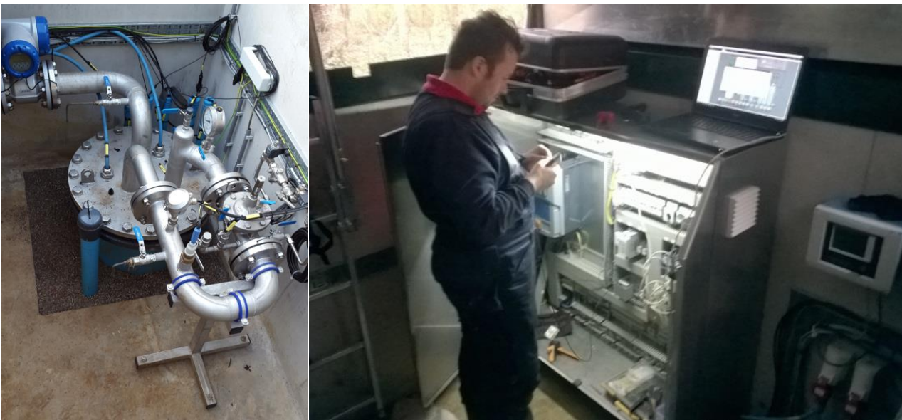
Figure 11: Left: Well chamber of the dedicated Freshkeeper. Right: John van der Klaauw (De Ruiter) is updating the control software in the well chamber.
