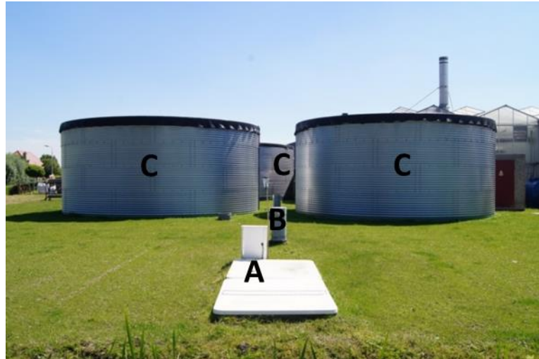
Figure 2-3 ASR-Coastal well field Nootdorp: infiltration well and monitoring equipment (A), monitoring wells (B) and storage tanks (C: one for rainwater, others for water reuse) (Zuurbier et al., 2014).
