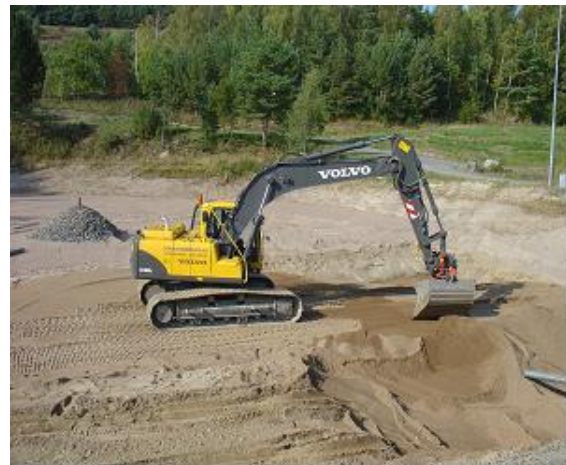
Figure 3: Excavator replacing slow filter sand after deep sand replacement at Dösebacka.
