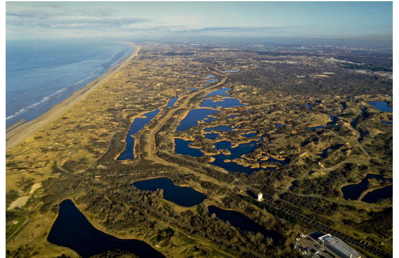
Surface water infiltration basins along the Dutch coast for treatment and storage of drinking water
