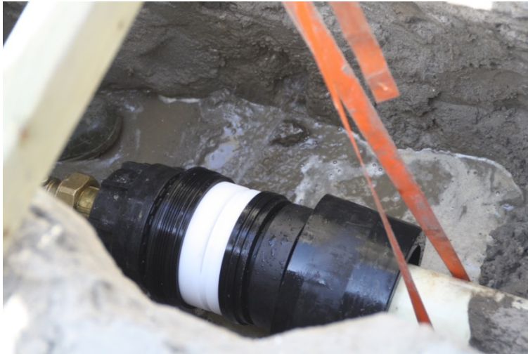
Figure 3.6 Lock joint with open cap (Photograph taken during pilot Dunea, 2015).
