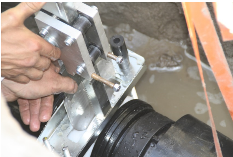
Figure 3.7 Inserting spade into Lock joint (Photograph taken during pilot Dunea, 2015).
