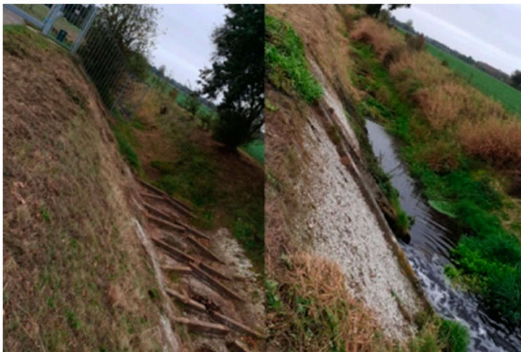
Figure A1. Discharge of TWW from the Haaksbergen WWTP into the Bolscherbeek (right) with dry stream bed shown upstream (left). Taken in drought conditions experienced in 2018.
