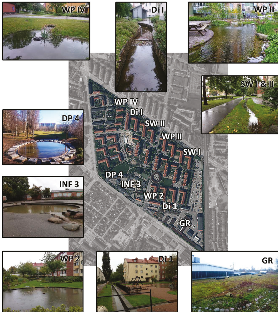
Figure A1. The photos of some of the implemented SCMs in Augustenborg. Different types of SCMs are shown in the figure as follows: (DP 4) dry pond, (Di I & 1) stormwater ditch, (SW I & II) swale, (WP 2, II & IV) wet pond, (INF 3) infiltration basin, (GR) green roof. The major runoff directions in the Northern and Southern systems are SW I → WP IV and GR → DP 4, respectively. Pictures for INF 3, WP 2, Di 1, and SW I & II are taken by Henrik Thorén (Rambøll). Background picture: GSD-Orthophoto, courtesy of The Swedish Mapping, Cadastral and Land Registration Authority, ©Lantmäteriet (2015).
