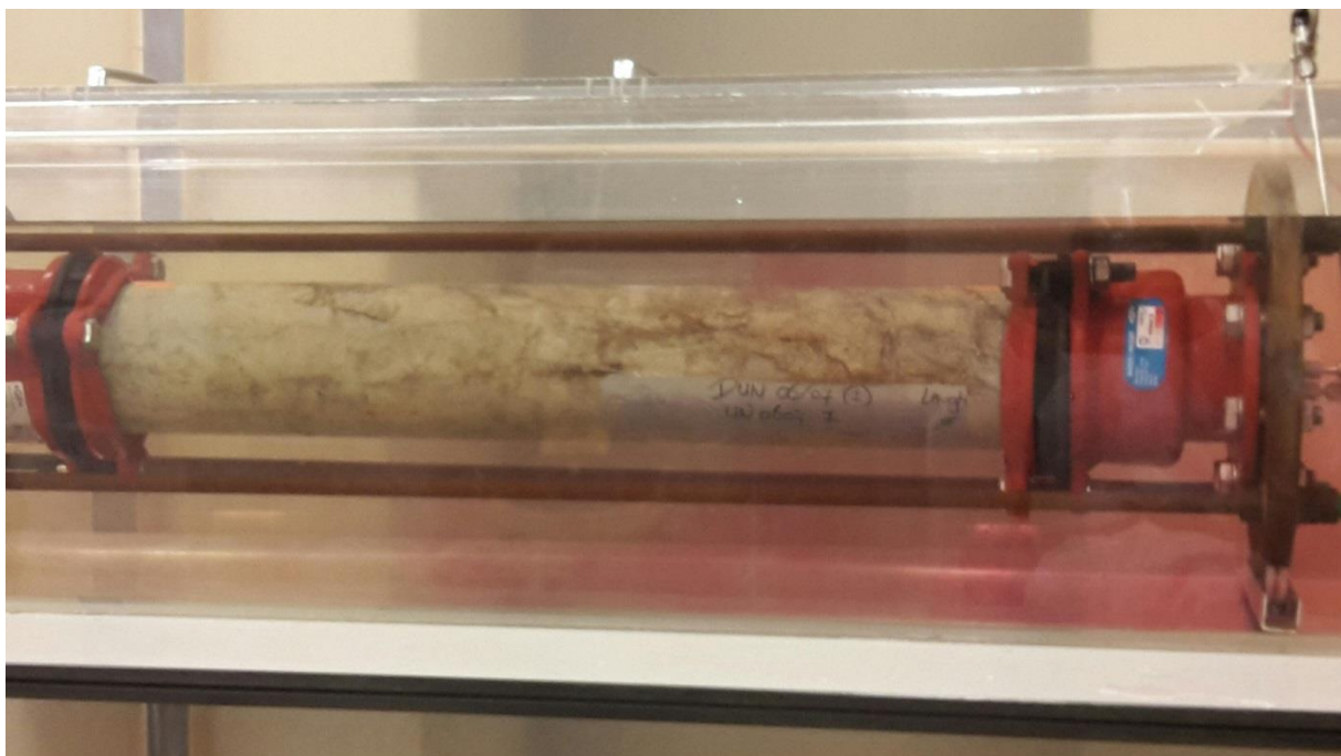
Figure 3.2.4.2: The leaching of the connected joint.
