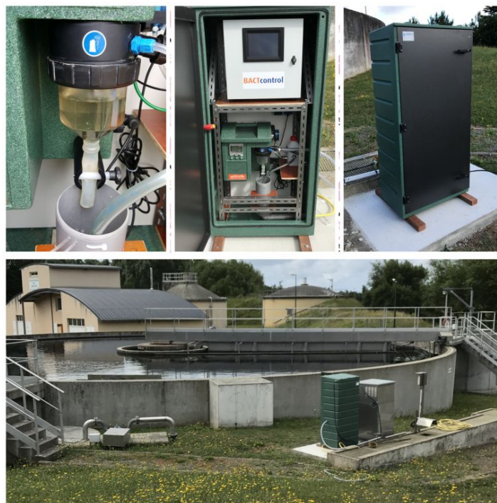
Figure 23 Test setup of the BACTcontrol at Agon Coutainville
