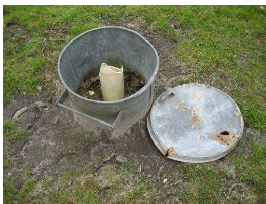
Figure 3.2 Unsealed abandoned observation well. Photo courtesy of KWR.
