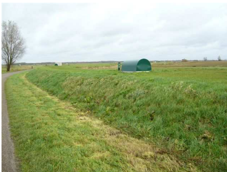
Figure 3.4. Water production well installed on top of a dike. The dike was newly constructed for this purpose, a flood preventive measure fitting in perfectly in the Dutch polder landscape. Photo courtesy of water supply company Groningen, the Netherlands
