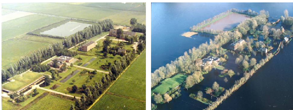
Figure 1.1. Pumping station Onnen (water supply company Groningen, the Netherlands), before (left) and after the 1998 flood (right).
