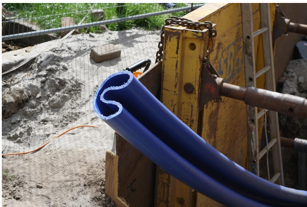
Figure 2 Application of Compact Pipe in Zwaagwesteinde, Friesland.
