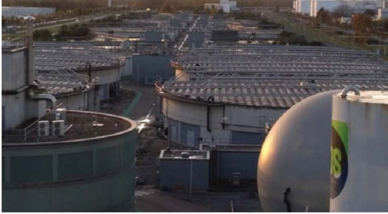
WWTP Amst erdam West (Source: fiware4water.eu)
