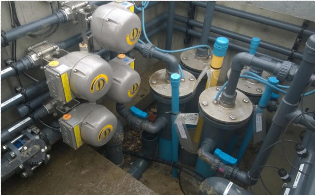
Multiple partially penetrating wells (MPPW)
