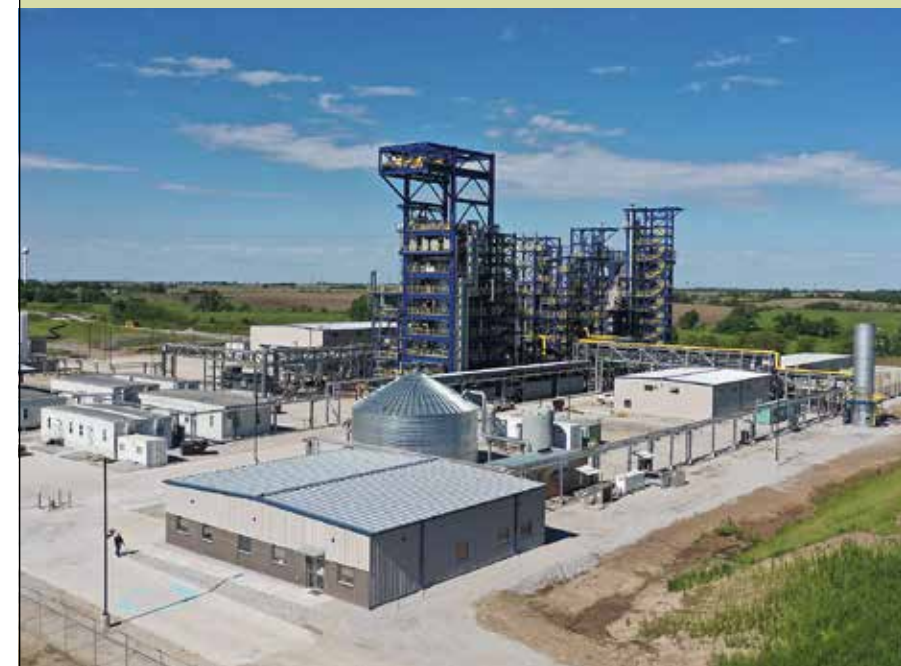
Monolith, methane pyrolysis plant in Nebraska, USA [145]
