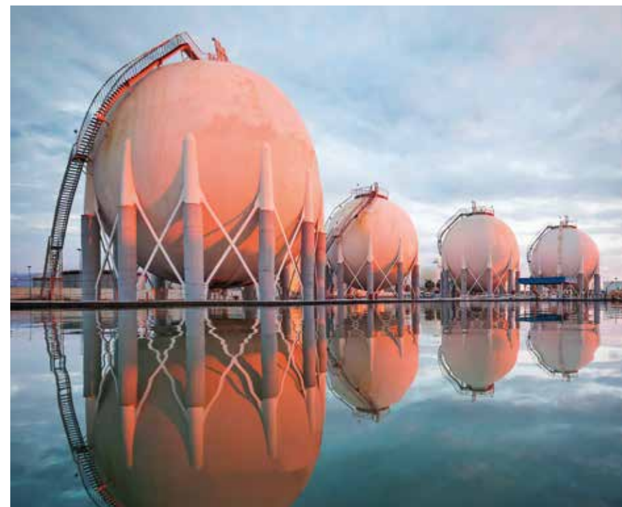
Spherical tanks for liquid-hydrogen storage
