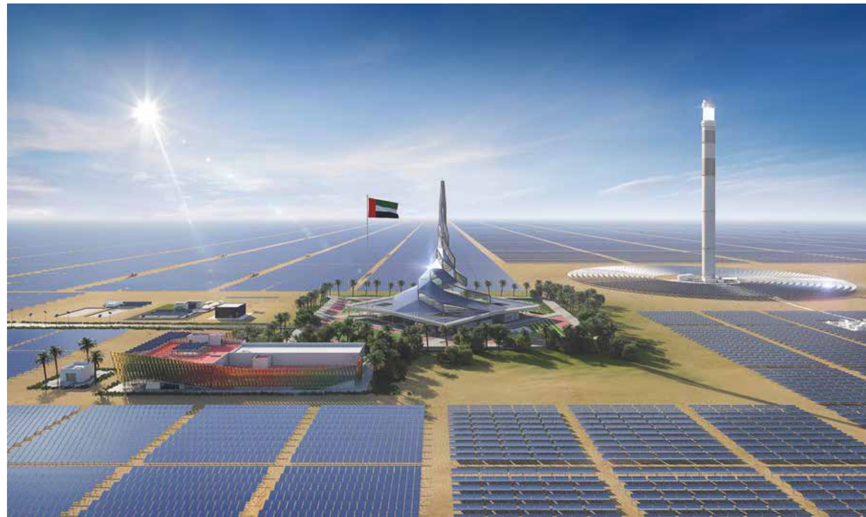
The Mohammed Bin Rashid Al Maktoum Solar Park in Dubai, with 3 GW of solar panels and CSP solar energy system [72]
