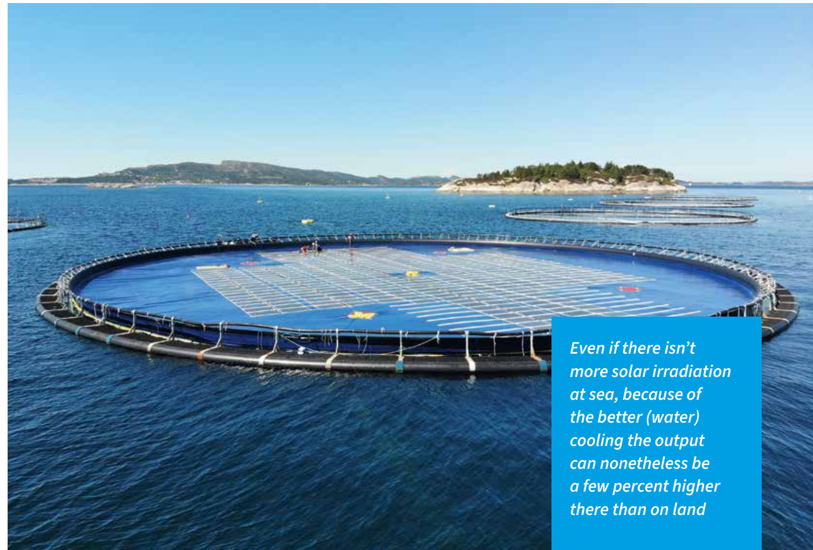
Floating solar panels on a hydro-elastic membrane, suited for application with high waves [107]
