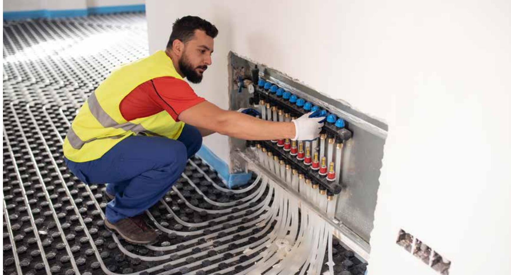
Installation of low-temperature heating
