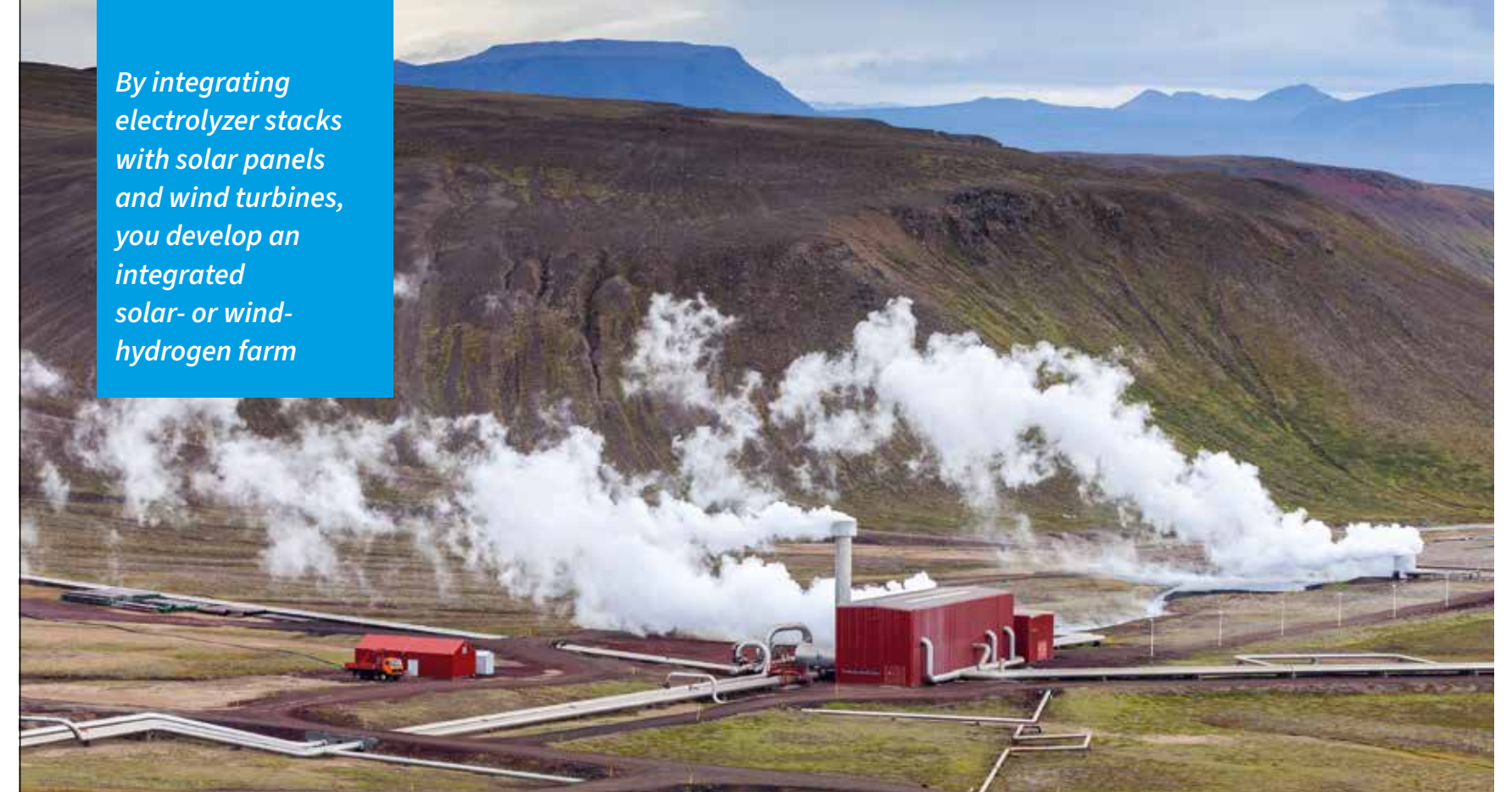
Geothermal power plant in Iceland
