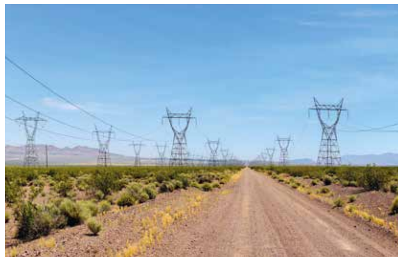
Electricity transport via high-voltage lines
