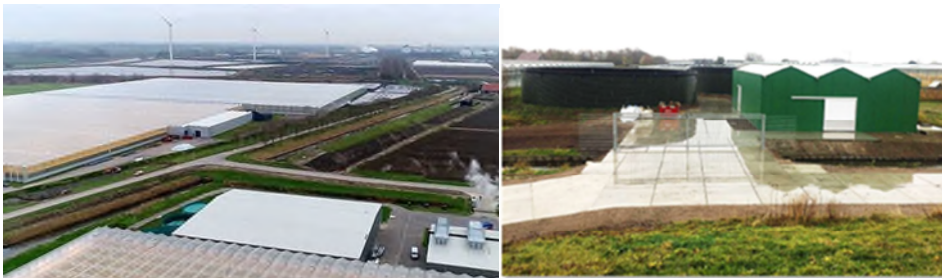
Figure 3. Greenhouse Horticulture in the Netherlands (left) and Wastewater Treatment Plant at De Vlot (right).
