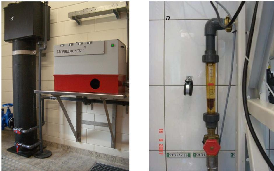
**Figure 3.1** Constant water flow to the MOSSELMONITOR®
