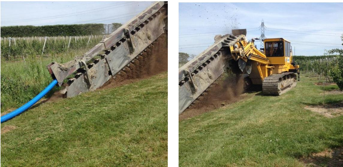
Figure 9.17: Installation of the 5 m deep drain to increase the freshwater recovery in Ovezande in June 2017
