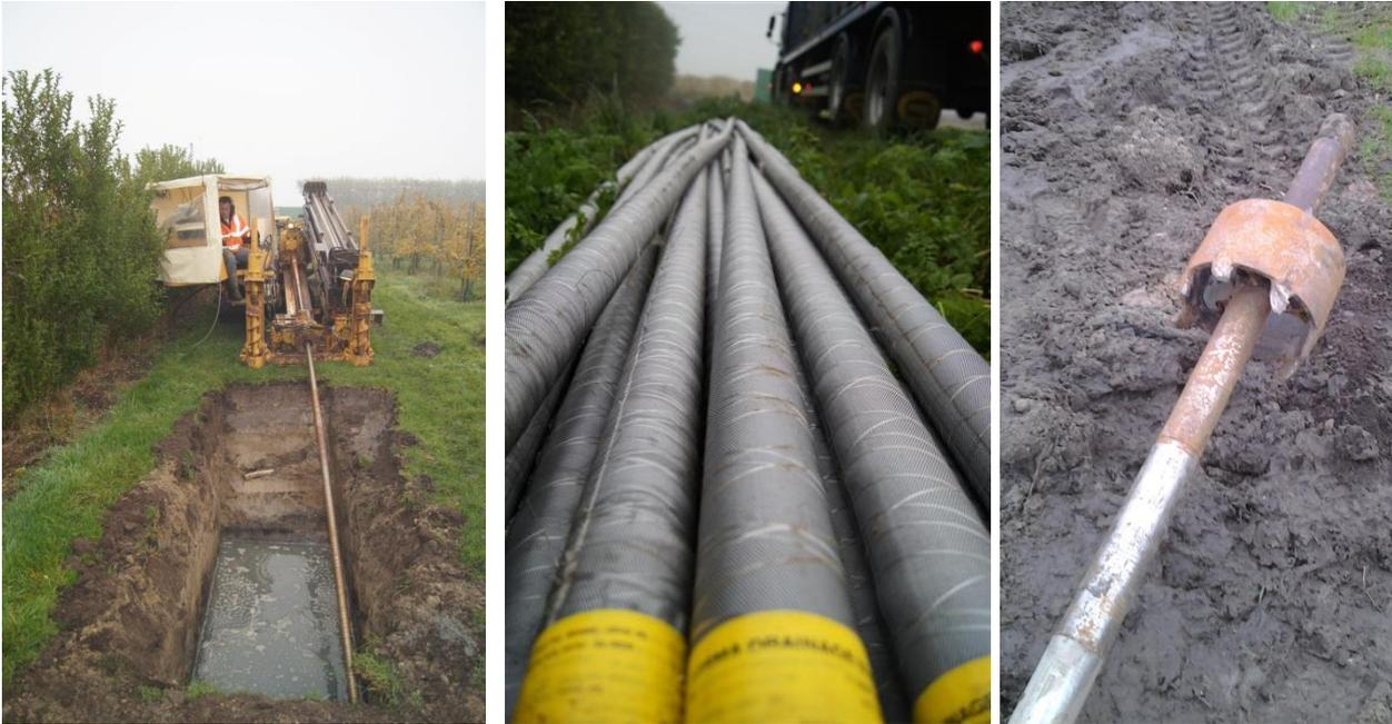
Figure 2.11: Drilling of the horizontal borehole (left) and the 75 mm HDPE well screens wrapped in geo-textile (middle) and the reamer used to create the 300 mm borehole (right)
