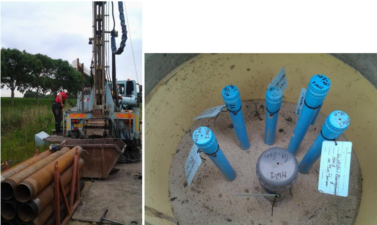
Figure 4-6: Drilling of the exploration well (left) and the resulting monitoring wells (right).
