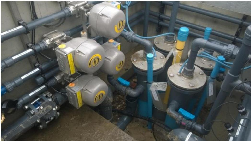
Figure 4-14: Realised ASR-Coastal well at Dinteloord, including supply and recovery lines and sensors.
