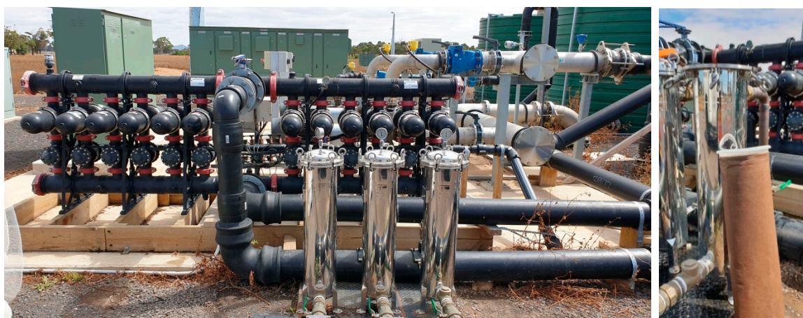
Figure 8. (Left): Central manifold ASR System with temporary prefiltration unit that includes a 20 \mu\text{m} spin Klin disc (the 12 black cylinders) followed by a 1 \mu\text{m} bag filter (the 3 upright cylinders). (Right): clogging of the 1 \mu\text{m} bag filter after ~2 days of operation.
