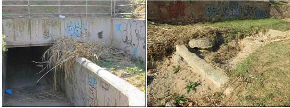
**Figure 45. Plenty sediment trap in the upper stream part of Canyadó’s catchment (Source: Advanced Mangement of Sediments in Sewers. Internal SUEZ R+D+i project)**
