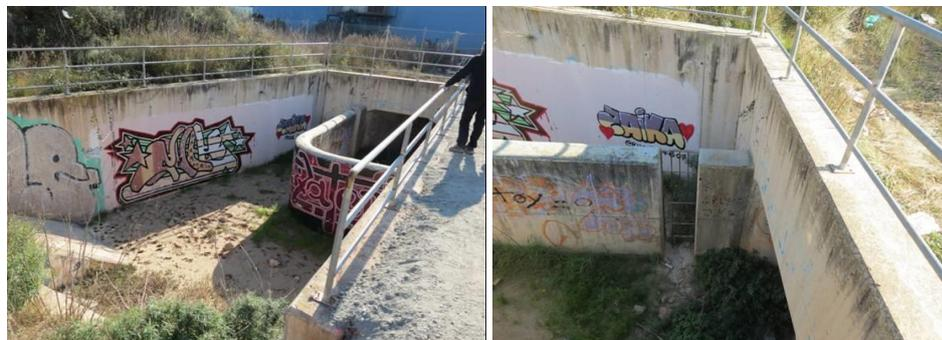
**Figure 44. Sediment trap in the upper stream part of Vallmajor's catchment (Source: Advanced Mangement of Sediments in Sewers. Internal SUEZ R+D+i project)**
