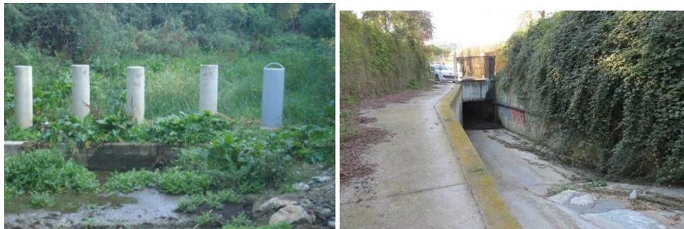
**Figure 43. Interceptors structures avoiding large objects and sediment trap in the upper stream part of Canyet's catchment (Source: Advanced Mangement of Sediments in Sewers. R+D+i Alliance)**
