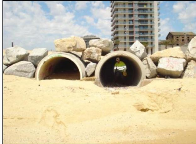
**Figure 49. Clogging phenomenon of the overflows infrastructures (Source Badalona DMP)**
