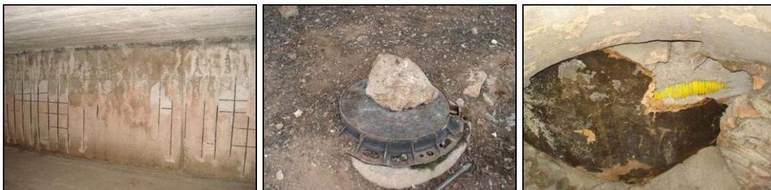
Figure 48. Material deterioration in the Badalona sewer network and some example of structural problems
