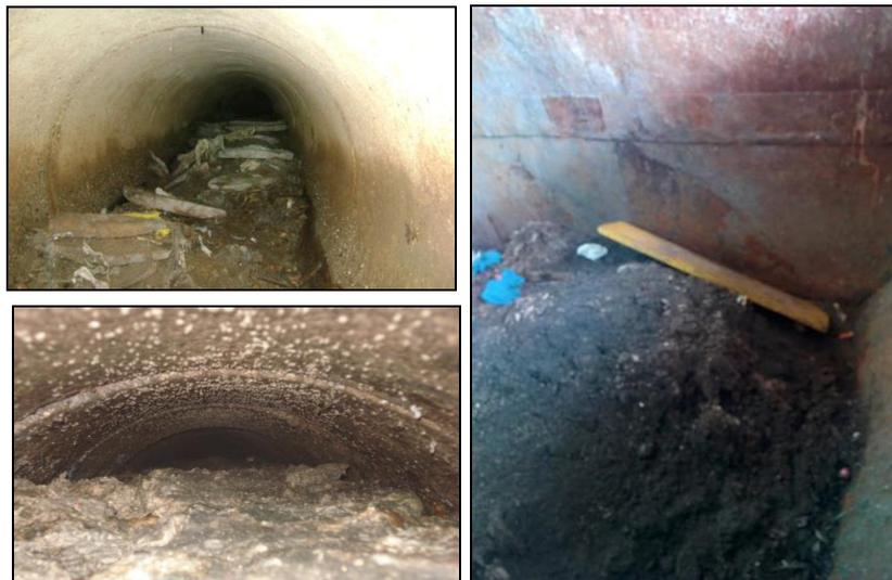
**Figure 46. Examples of sediments within Badalona’s sewer network (right) and the deposits extracted at the Badalona Harbour pumping station (left)**
