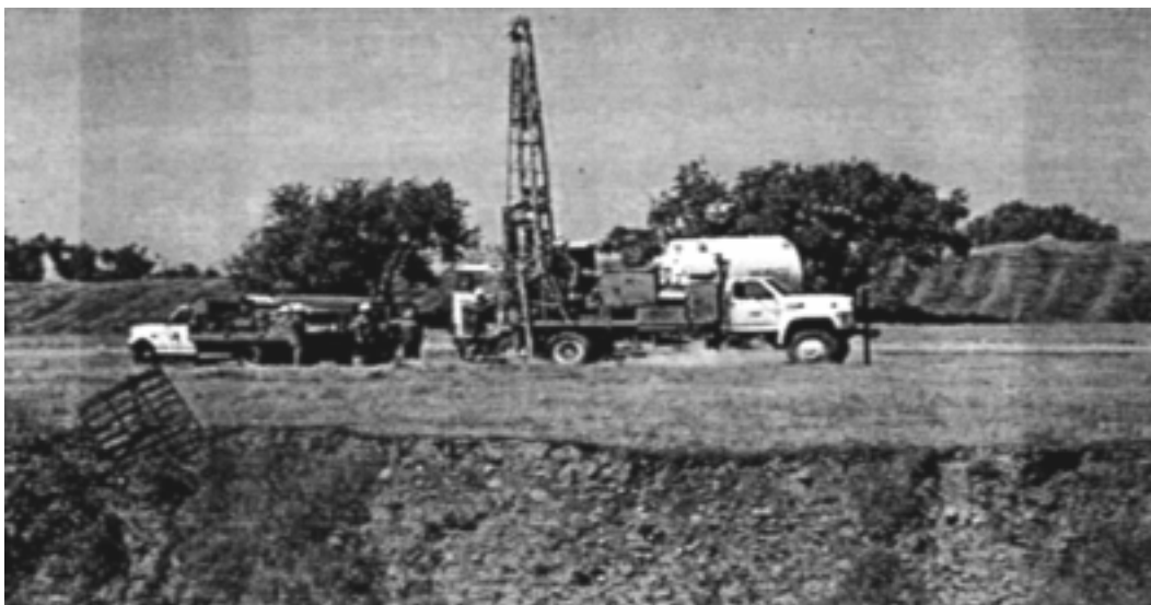
Figure 6. A cryogenic drilling site. Large boulders in the subsurface, visibly exposed in the trench in the foreground, do not present a drilling challenge using this technique.
