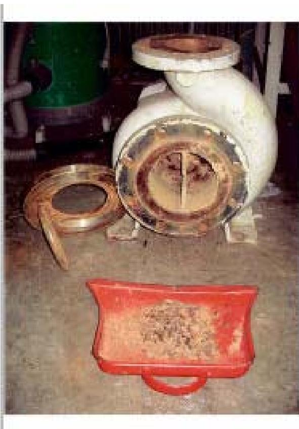
**Figure 6-1. Iron sediments from the pump station Vierlingsbeek.**
