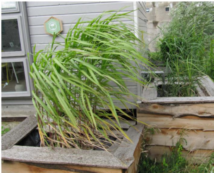
FIGURE 1 INDIVIDUAL BIOFILTER (2 TANKS) FOR GREY WATER TREATMENT
