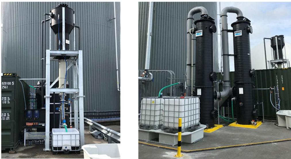
Figure 53. CS7: Photos of the struvite reactor (left) and ammonia stripping units (right).
